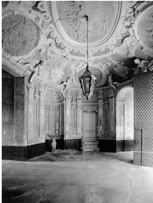
4. Atrium of palazzo Nicolosio Lomellino in Genoa, before restoration.
